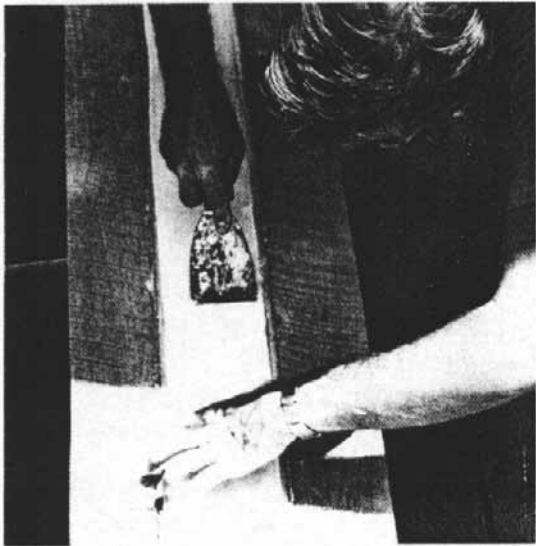
FIGURE 4.10—Smoothing out a new layer of silicone over the cloth, completely embedding the cloth (Skyheat Workshop photo).
