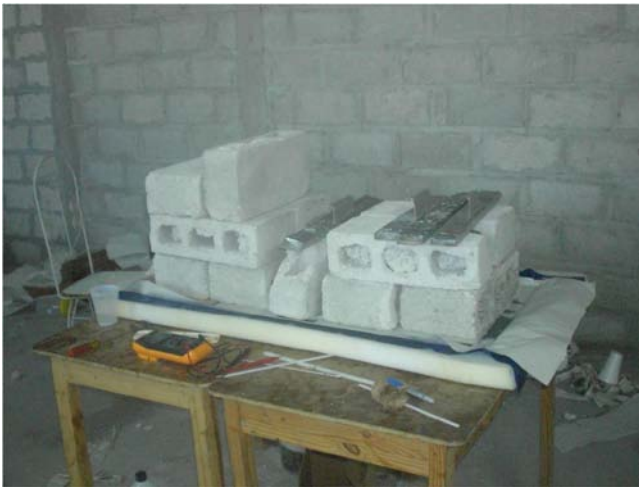
Fig 5 Low-tech laminating system using heavy weights, developed by Enersa in Haiti.
